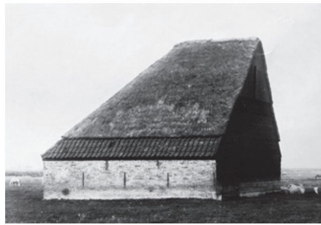
A barn for sheep with a clear layering of materials; bricks, roof tiles and reed.
